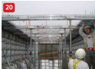
Setting Slab Soffit Incorners
