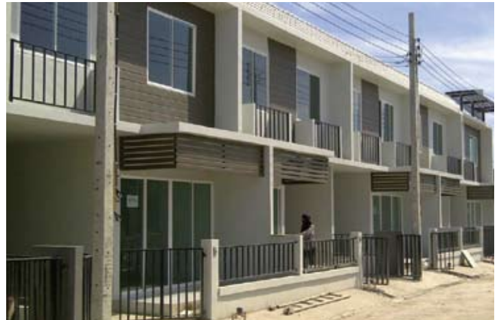
06 PROJECT NAME : The Colors Townhouses Country : Thailand CONSTRUCTION TYPE : Aluminum Formwork
