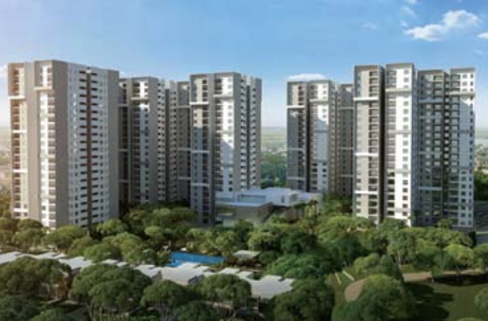
36 PROJECT NAME: Silicon Oasis Country: India CONSTRUCTION TYPE: Aluminum Formwork
