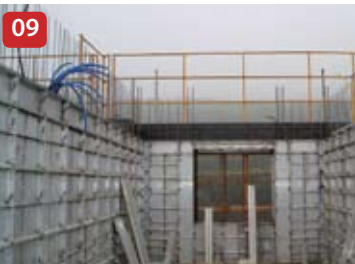
Setting Wall Panels
