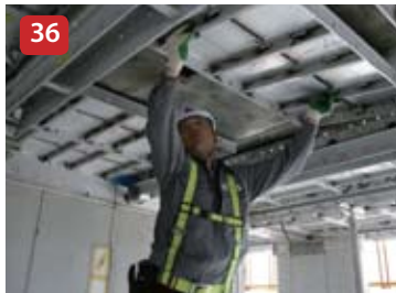
Dismantling from Slab to Wall Panels in sequence
