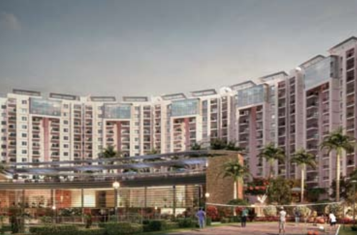
32 PROJECT NAME: Lakefront Country: India CONSTRUCTION TYPE: Aluminum Formwork
