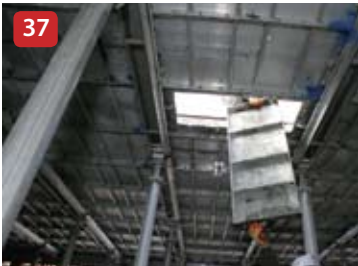
Lifting forms to next level
