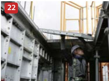
Setting Slab Panels
