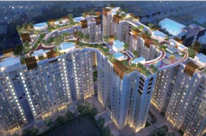
31 PROJECT NAME: Suburbia Country: India CONSTRUCTION TYPE: Aluminum Formwork
