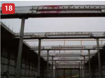
Setting Slab Beams
