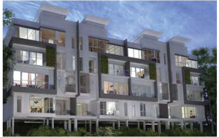
02 PROJECT NAME : Sunway Montana Country : Malaysia CONSTRUCTION TYPE : Aluminum Formwork
