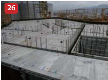
Setting Slab Panels
