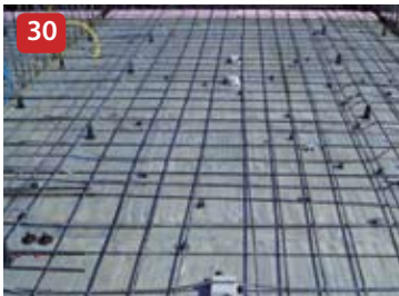
Setting Rebars on slab
