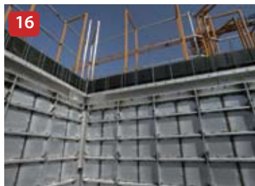
Setting Slab Soffit Incorners
