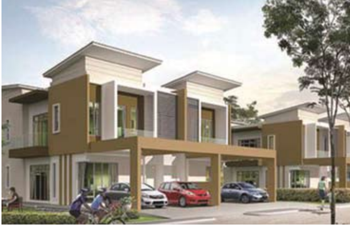
01 PROJECT NAME : Taman Pulasan 5 Housing Country : Malaysia CONSTRUCTION TYPE : Aluminum Formwork
