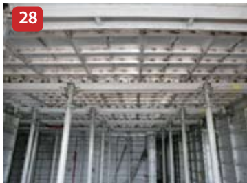
Slab Level Fine-Tuning
