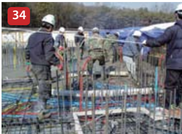
Setting Rebars on slab
