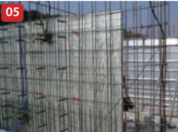
Setting Wall Panels
