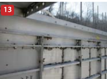
Setting Slab Soffit Length
