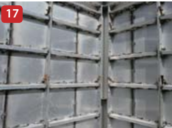
Setting Slab Soffit Incorners
