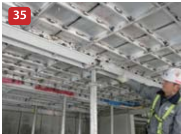
Dismantling from Slab to Wall Panels in sequence
