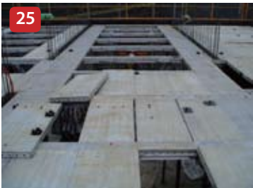
Setting Slab Panels
