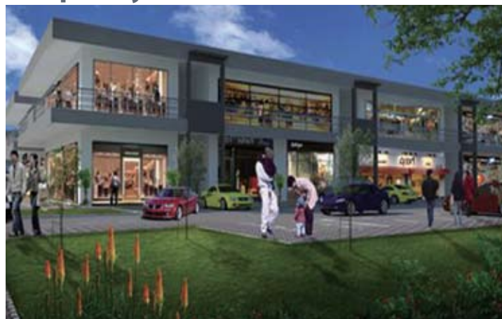
03 PROJECT NAME: Telupid Jaya Commercial Centre Country: Malaysia CONSTRUCTION TYPE: Aluminum Formwork
