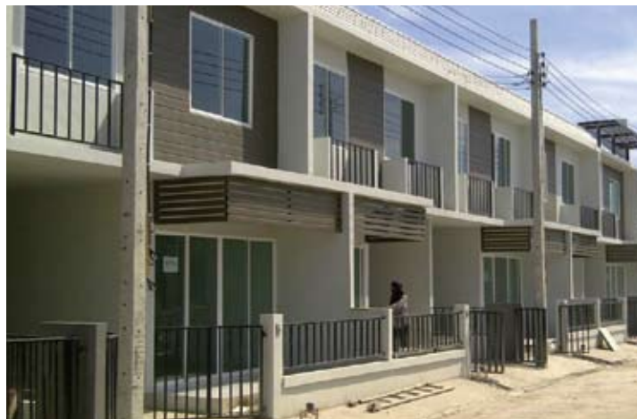
06 PROJECT NAME: The Colors Townhouses Country: Thailand CONSTRUCTION TYPE: Aluminum Formwork
